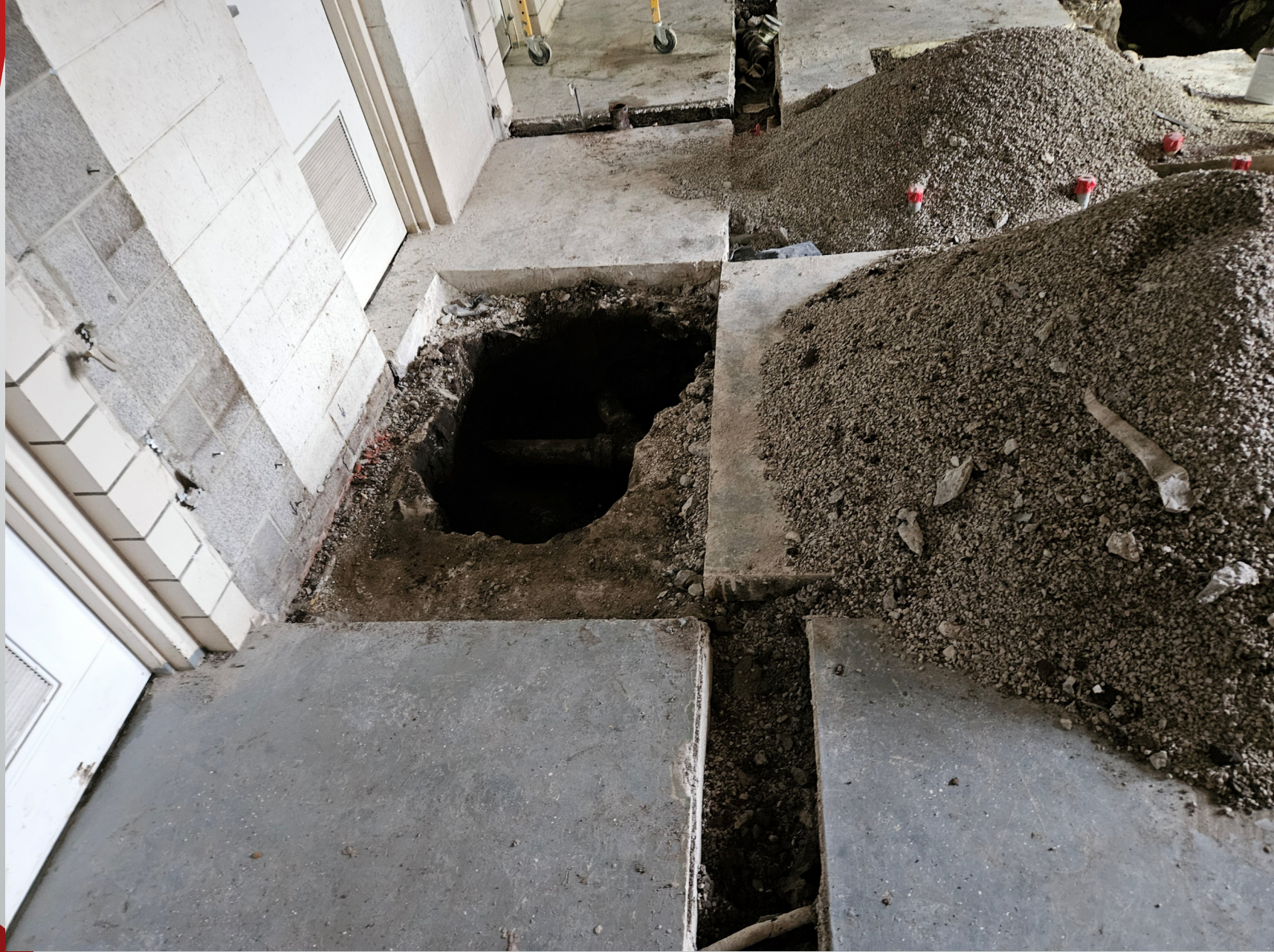
High School bathroom demolition completed and starting underground rough-in
