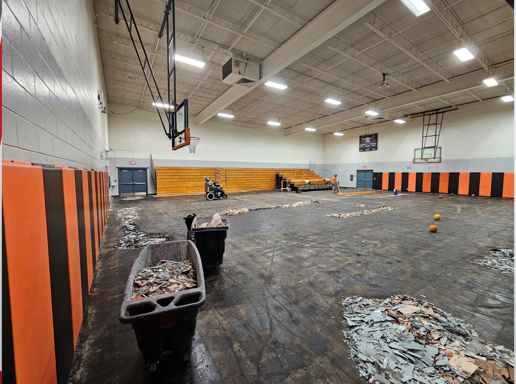
Bleacher and floor demolition at Elementary School gym.
