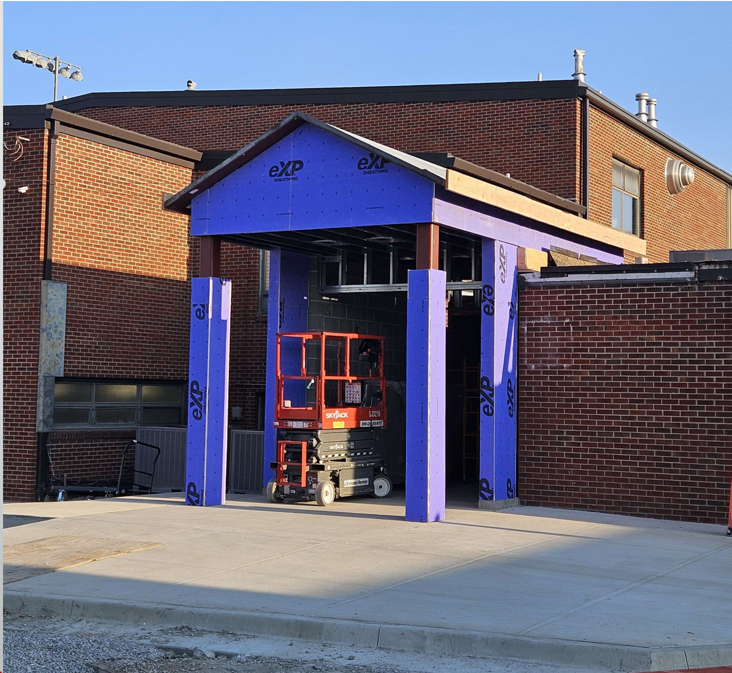
Metal roof deck and exterior sheathing installed for new High School Entrance
