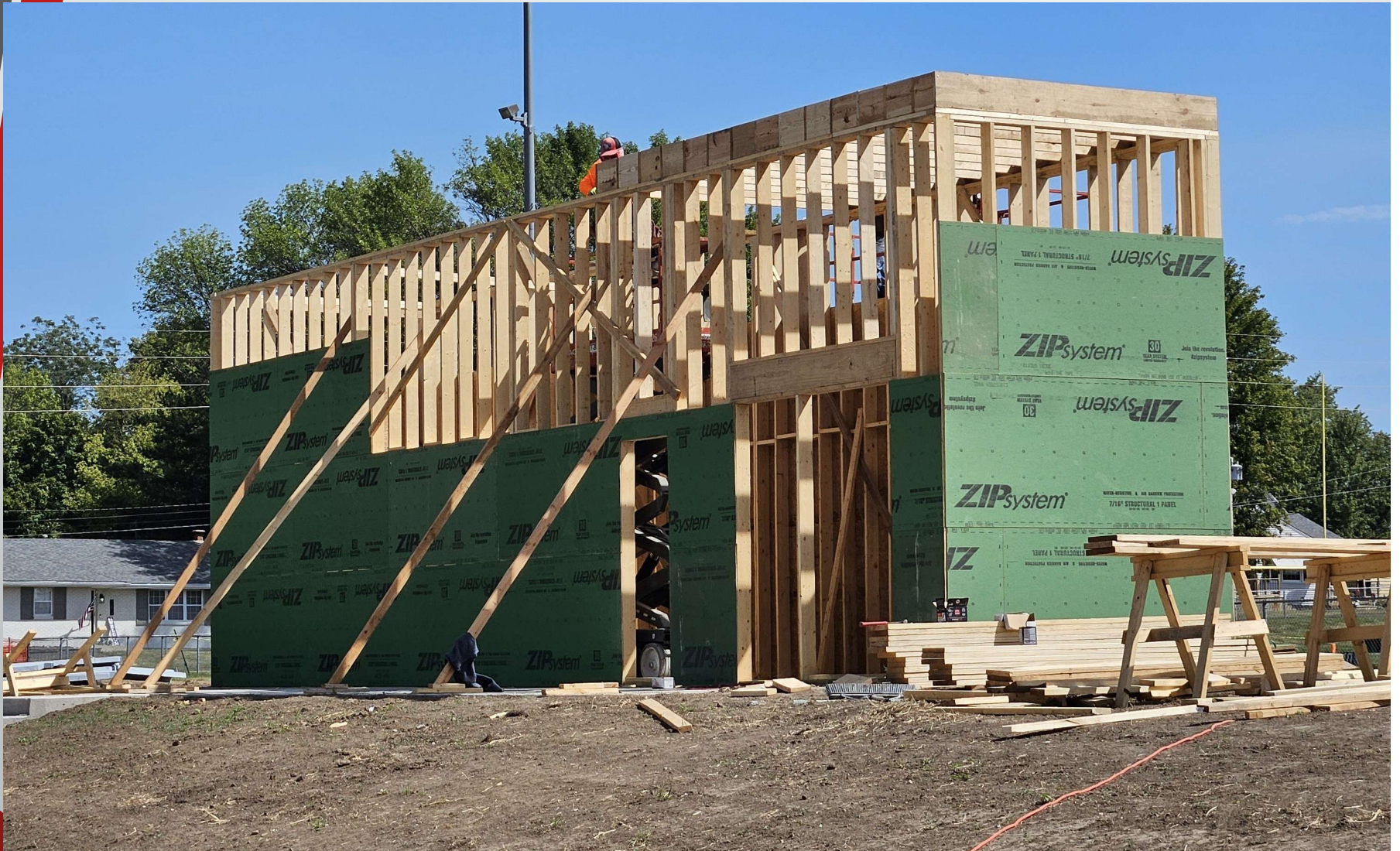
High School press box exterior framing
